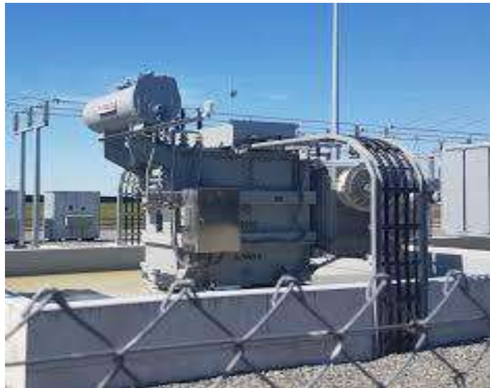
Fig 4.3 plinth mounted substation
